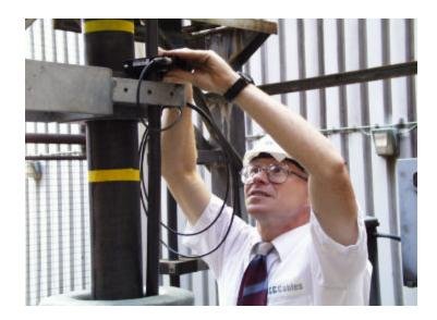
Figure 4 – Technician installing sensor on 138KV cable shield
