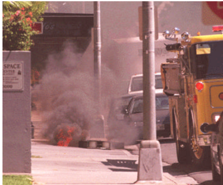
Fire comes from a manhole on Richards Street this morning.
